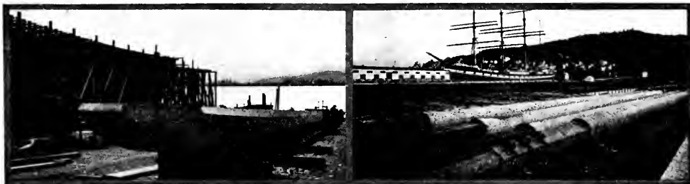
Two views at the McEachern Ship Company plant. Left, keel timber. Right, completed masts.
